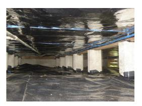
Thick polythene sheeting is available at most hardware stores. It is usually cut into strips (around 2 metres) and laid between the piles under the house. Slits are cut along one side of the strips to fit them around the piles and both the slits and the overlaps between strips are taped closed with polythene tape.
