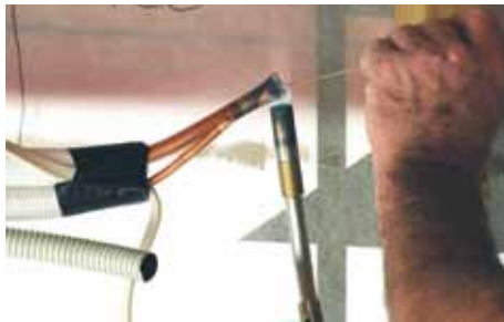
Figure 6.22 Braze pipe ends closed
