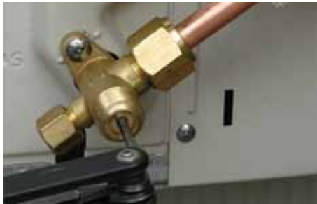
Figure 7.32 Progressively release the vacuum
