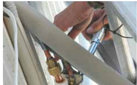
Figure 6.16 Tighten connection (B)
