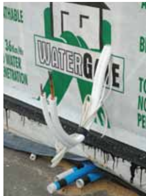
Figure 4.11 Pre-install pipework before building claddings are installed
