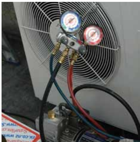
Figure 7.30 Remove vacuum pump and gauges (B)
