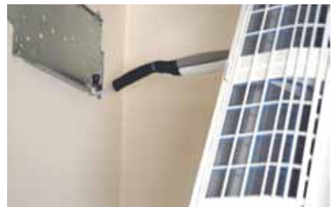
Figure 7.8 Feed taped bundle through the hole
