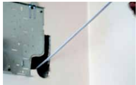
Figure 7.6 Feed the connecting cable through the wall
