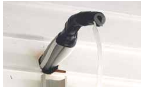
Figure 7.12 Taped pipes, drainage pipe and connection cable through hole
