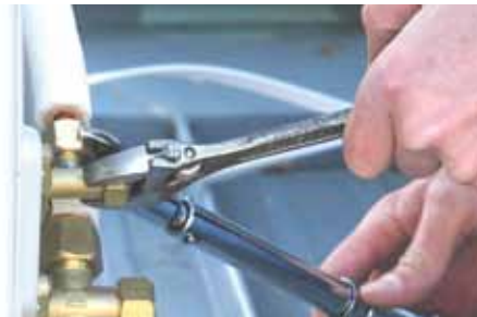
Figure 6.15 Tighten connection (A)
