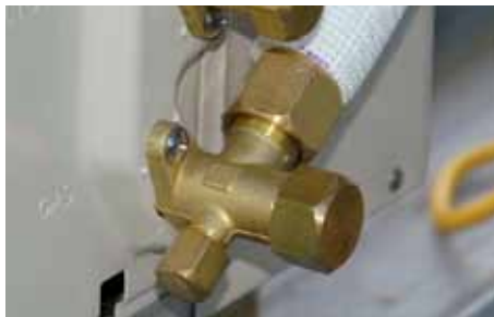
Figure 7.33 Tighten valve caps
