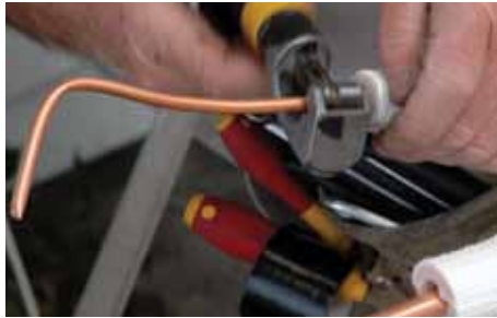
Figure 6.5 Cut pipe with tube cutters
