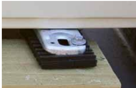
Figure 7.17 Pack with plastic shims to level
