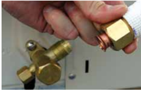
Figure 6.13 Connect the pipes (A)
