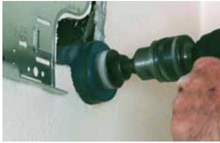
Figure 7.3 Drill a hole through the wall
