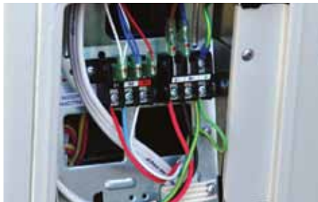
Figure 9.1 Connect power supply cable to terminal block
