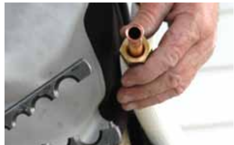
Figure 6.10 Flare the end of the tube (C)
