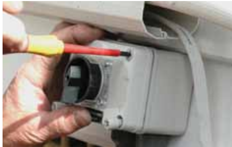
Figure 9.4 Install lockable isolating switch (C)
