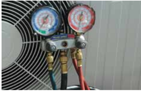
Figure 7.31 Remove vacuum pump and gauges (C)
