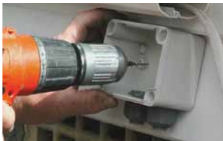
Figure 9.2 Install lockable isolating switch (A)
