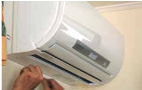
Figure 7.11 Ensure unit is securely seated
