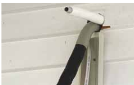
Figure 7.19 Bind insulation with vinyl tape
