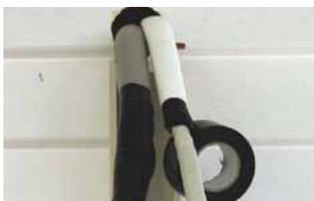
Figure 7.20 Tape drainage hose to drainage outlet
