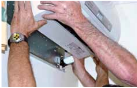
Figure 7.9 Attach unit to wall bracket (A)
