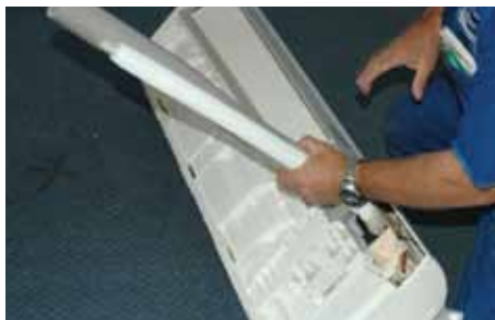
Figure 7.5 Release the tubing and drainage hose
