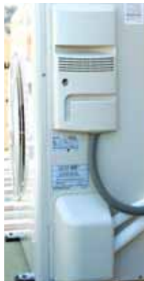
Figure 9.5 Replace service cover to outdoor unit
