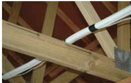
Figure 6.17 Run pipe/cable across truss chord/ceiling joist
