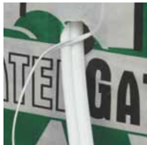
Figure 6.24 Feed pipe/cables through building wrap
