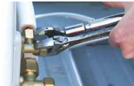
Figure 7.28 Tighten flare nut connections
