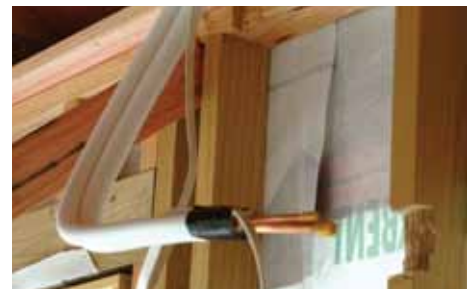
Figure 6.19 Notch the top plate and studs (B)
