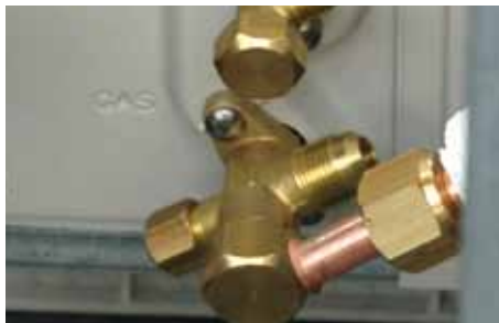
Figure 7.27 Connect pipes and tighten flare nut
