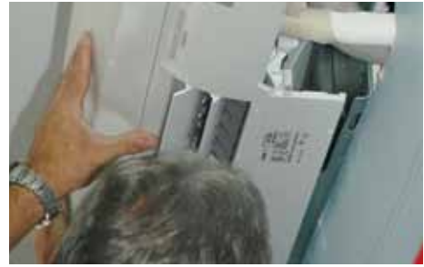
Figure 7.10 Attach unit to wall bracket (B)
