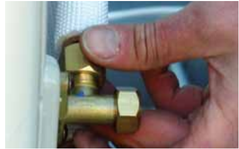
Figure 6.14 Connect the pipes (B)
