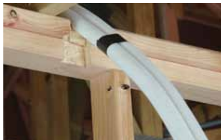
Figure 6.18 Notch the top plate and studs (A)
