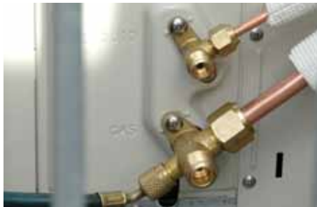
Figure 7.30 Remove vacuum pump and gauges (B)
