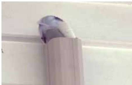
Figure 7.23 Fill hole around piping with sealant
