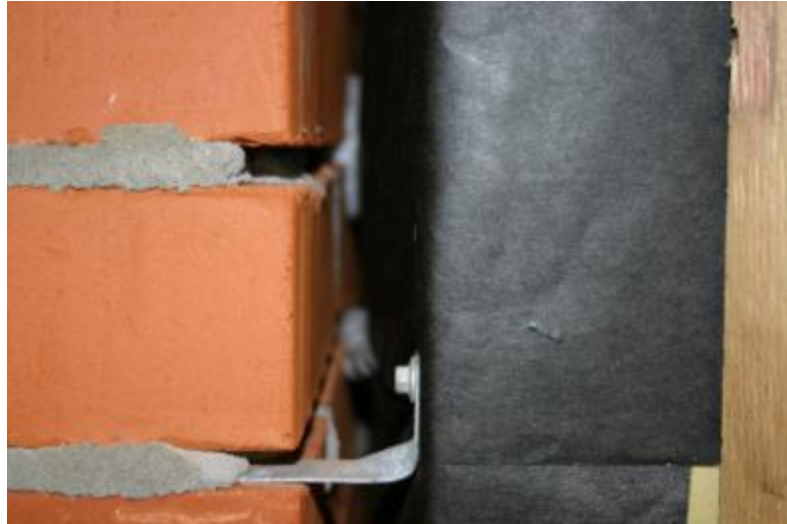
Figure 22: Cavity of Brick Veneer Wall (D4863a)
