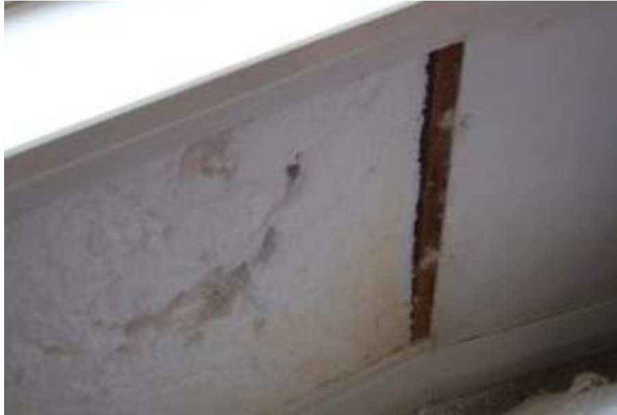
Figure 10: Removal of wallboard to assess Airfoam installation – note voids present house (House W3)
